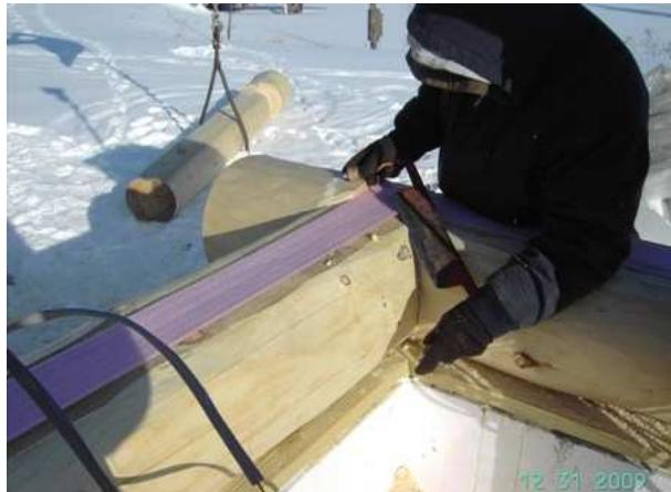
I like to touch-up the miters with a sander/grinder so that the edges meet.
