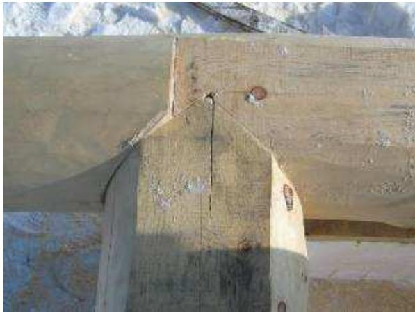
Next set the next passing log with the natural tail up on equal size blocks about 3 or 4 inches high. Be sure and line it up right where you want it and remember to hold the tail in slightly like the first log.
