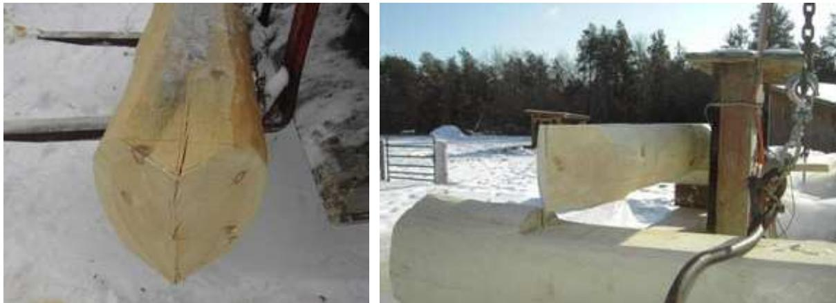
Then set the butting log with the point so that it is setting level onto the log with the natural tail (the passing log) and check to see if the two outer points line up with each other. Sometimes you will have to adjust the angle on one side of the point that you just cut so that they line up especially when the log below has a flare and is wider on one side than the other. Then trace it on the log below and cut it out and fit if necessary.
