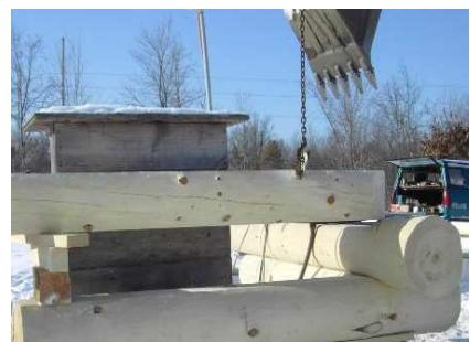
Next I like to match the edges so I trace the log and drawknife the wood off and round it some. You can also use a sander / grinder or chainsaw. I like to finish it up with the drawknife because it closes the pores in the wood and the stain matches better.
