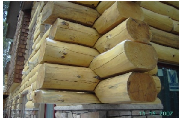
Hand-Peeled 10" Double Round flat on flat with saddle notch option
