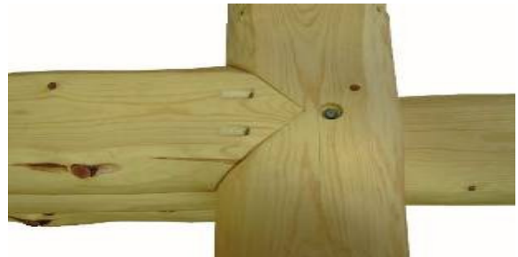
Top view of butt and pass notch
