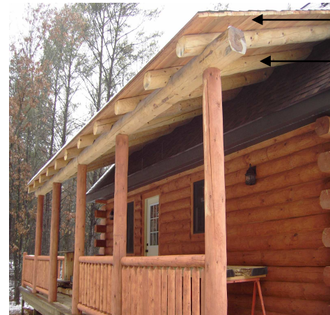
2 x 8 T&G Log rafters
